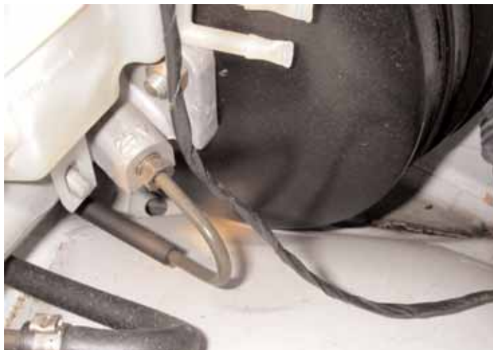
Photo #3 Drain Hole Under Master Cylinder And Booster
