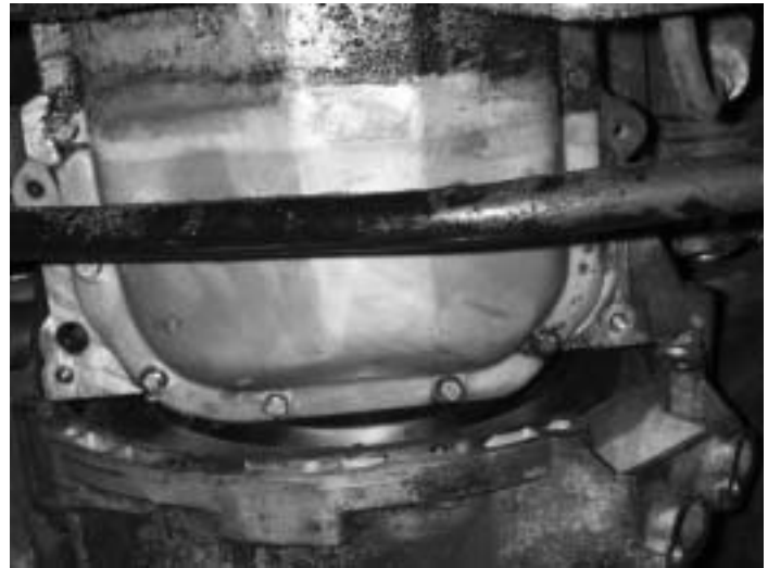
Photo #2 Oil-Pan Bolts Exposed.
