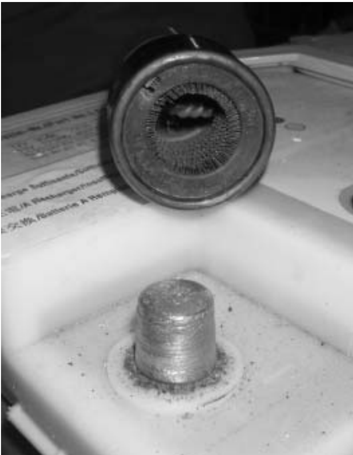
Photo #2 Shiny surface on battery post
