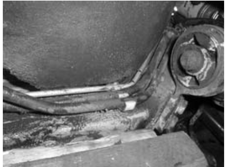
Photo #4 New Tubing Installed
